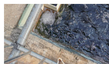
Sewage Treatment Plant
