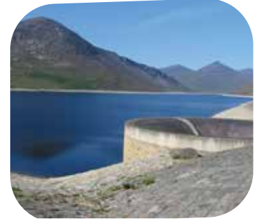
Raw water monitoring of water works
