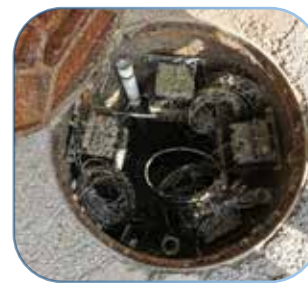
Urban domestic sewage monitoring
